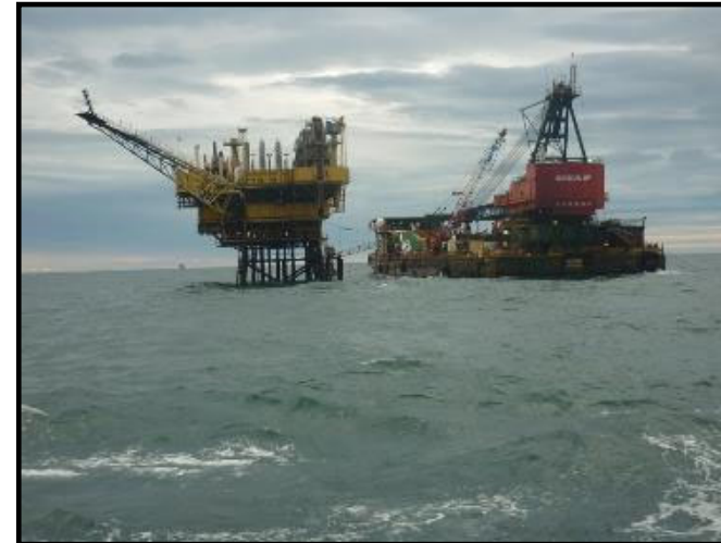
Repair AM2 platform production
